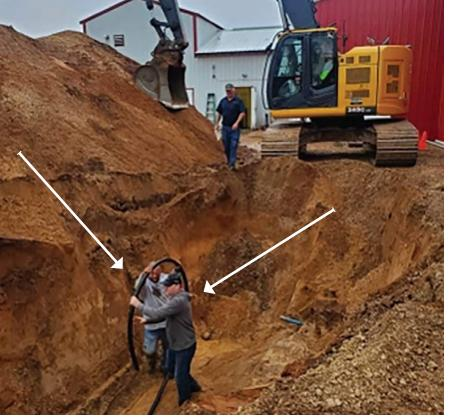
Hydraulic Shoring works by the shores (cylinders) pushing against the trench face using hydraulic (fluid) pressure. The pressure created between the two cylinders creates an arching effect that will hold back the side walls of the trench. The workers must work between the cylinders.
