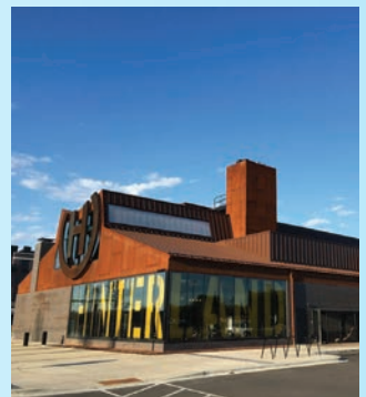
Hinterland Brewery HVAC and Plumbing Insulation, Performance Firestop, Inc.
