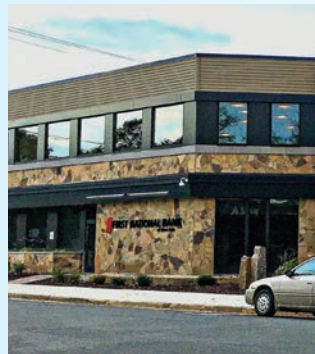
First National Bank of River Falls, Derrick Companies
