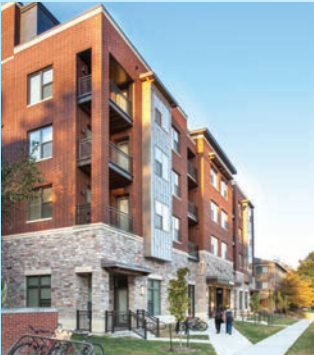
Whistler Student Apartments, Stevens Construction Corp.
