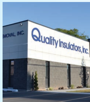
Quality Insulators, Inc., Keller, Inc.
