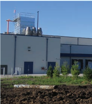
Greenfield Refrigerated Warehouse Facility, ESI Constructors, Inc.
