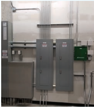
W.D.S. Construction, Inc. Headquarters, Steiner Electric, Inc.
