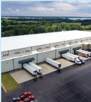
Beaver Dam Cold Storage, WDS Construction, Inc.
