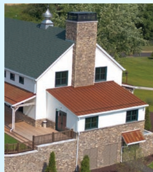
Harvest Haven Barn, National Construction
