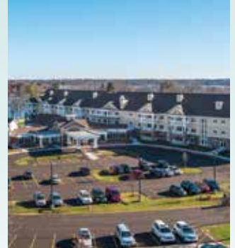
Shorehaven Health Center-Wellness Residences / Altius Building Company
