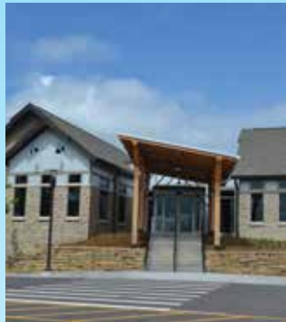
Gordon Bubolz Nature Preserve - Environmental Center and Microgrid / Faith Technologies, Inc.
