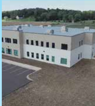
St. Croix Valley Business Innovation Center / Ross & Associates, Ltd.
