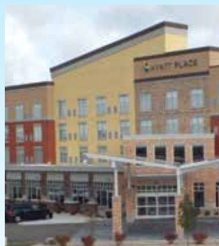
Hyatt Place Hotel KSW Construction
