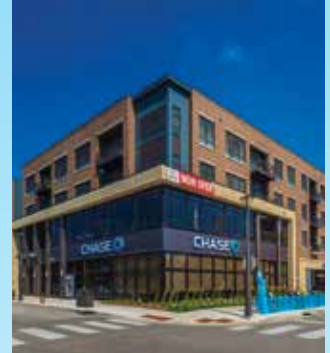
State Street Station Stevens Construction Corp.
