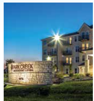
Park Creek Independent Living Consolidated Construction Co., Inc.
