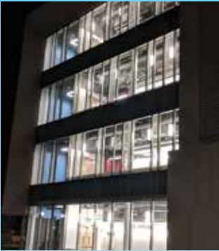
UW LaCrosse New Science Lab Building / North American Mechanical, Inc.
