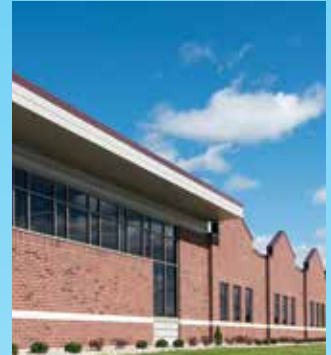
Fox Valley Lutheran High School Catalyst Construction
