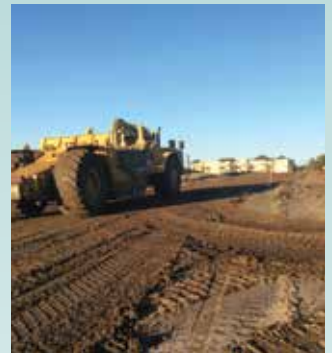
Kalahari Resort Conference Center Sitework / Friede & Associates
