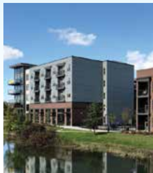
The Marling Stevens Construction Corp.
