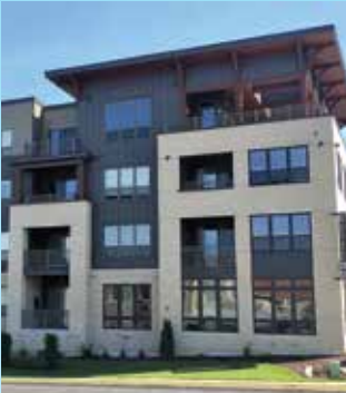
Watts Hill Apartments McGann Construction, Inc.
