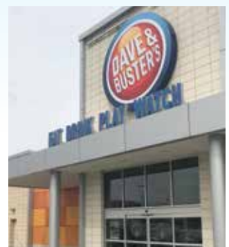
Dave & Buster's WDS Construction, Inc.
