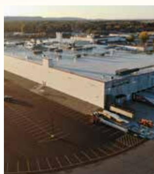
Kwik Trip Bakery - Bread/Bun Line Production Facility / Wieser Brothers
