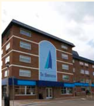
Harborview Hotel Remodel Northcentral Construction
