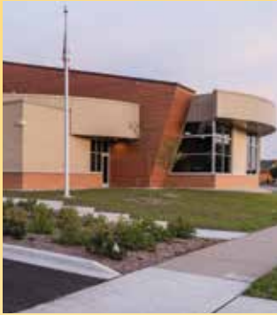
School District of Beloit New Welcome Center / Gilbank Construction, Inc.
