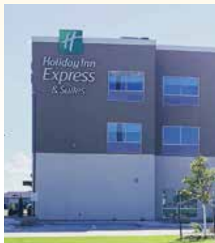
Holiday Inn Express & Suites WDS Construction, Inc.
