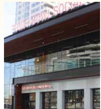
Punch Bowl Social WDS Construction, Inc.
