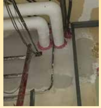
Milwaukee City Hall 3rd floor renovation / Alpha Insulation and Waterproofing, Inc.
