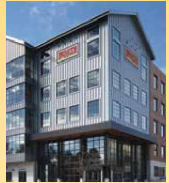
Duluth Trading Company Corporate Headquarters / National Construction
