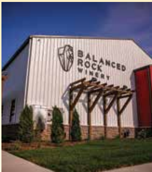
Balanced Rock Winery Friede & Associates
