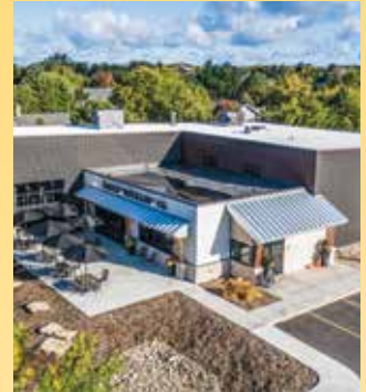
Hatch Distilling Company Keller, Inc.
