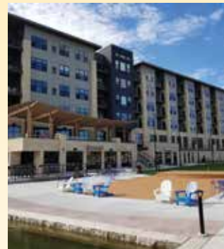
The Current McGann Construction
