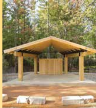
Schmeckle Reserve - Amphitheater Development / Ellis Construction
