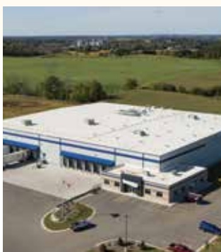
Cedar Valley Cheese WDS Construction, Inc.
