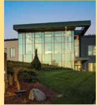
Illumina - New Research Facility Faith Technologies, Inc.
