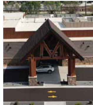
Mineshaft Keller, Inc.
