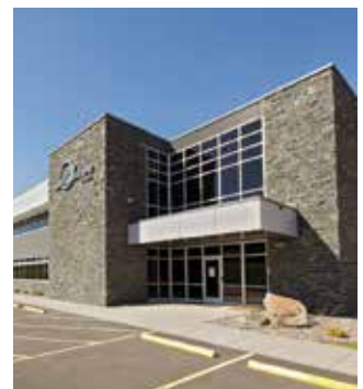
AROW Global Office Expansion Ellis Construction
