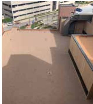
UWHC Clinical Science Center Pioneer Roofing, LLC
