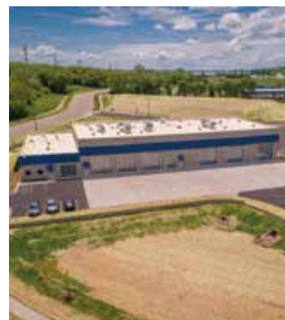
Certco Fleet Maintenance Facility Stevens Construction Corp.
