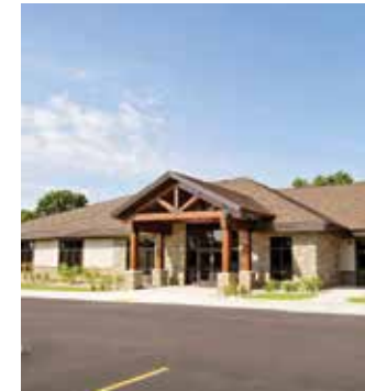
Mt. Morris Mutual Insurance Company New Headquarters Ellis Construction
