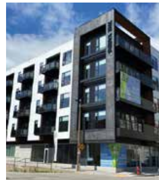
The Yards Altius Building Company
