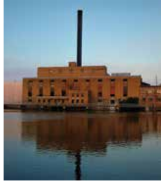
Beloit College Powerhouse Corporate Contractors Inc.
