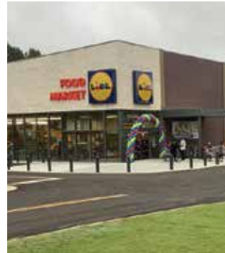
LIDL Grocery WDS Construction, Inc.
