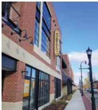
The Lamphouse McGann Construction
