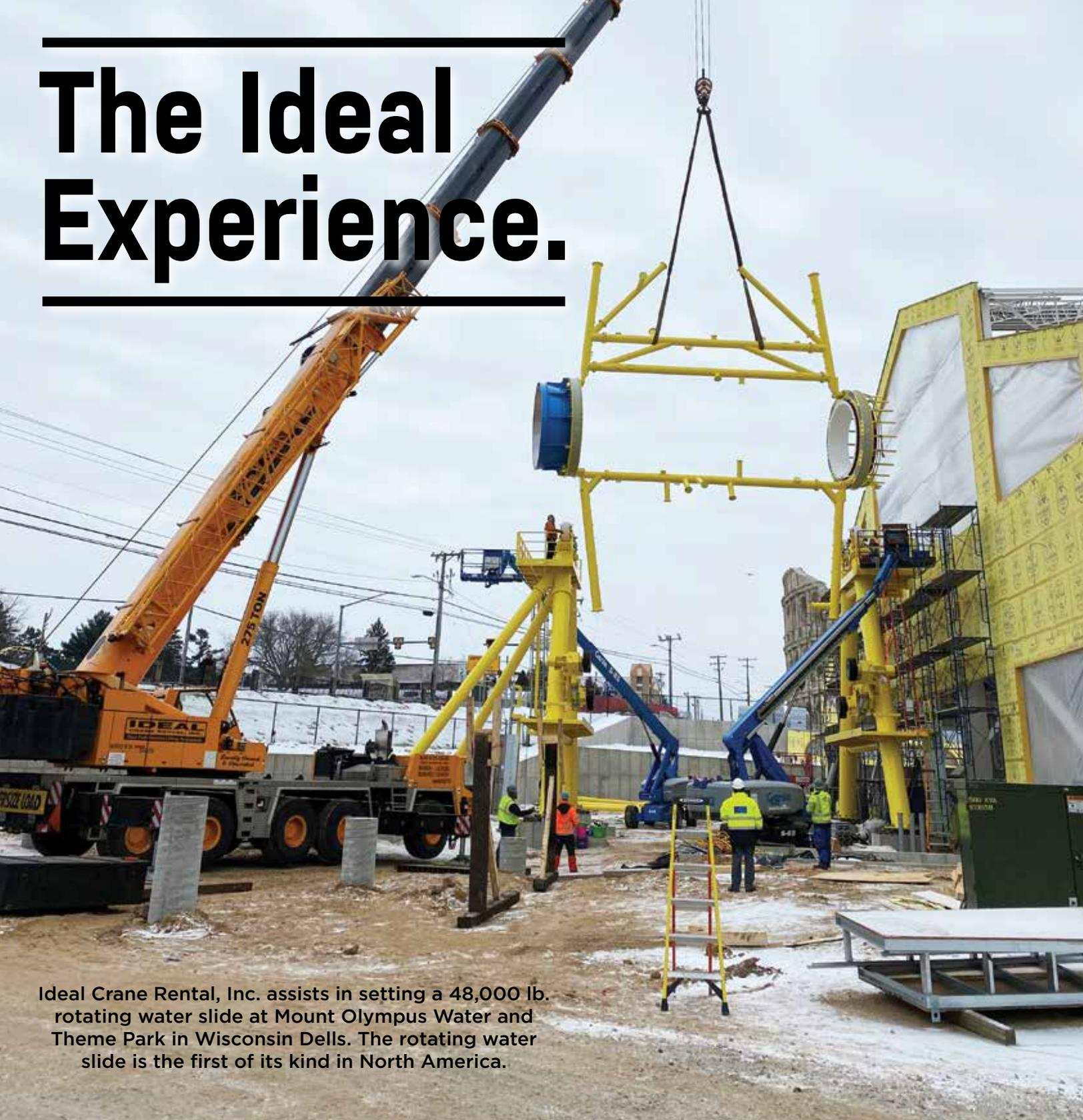
A large yellow crane is lifting a massive yellow metal structure, likely a rotating water slide, at a construction site. The structure is suspended by cables and is being positioned near a building under construction. Several workers in safety gear are visible on the ground and on the structure. The scene is set in a construction area with a dirt and snow-covered ground.
